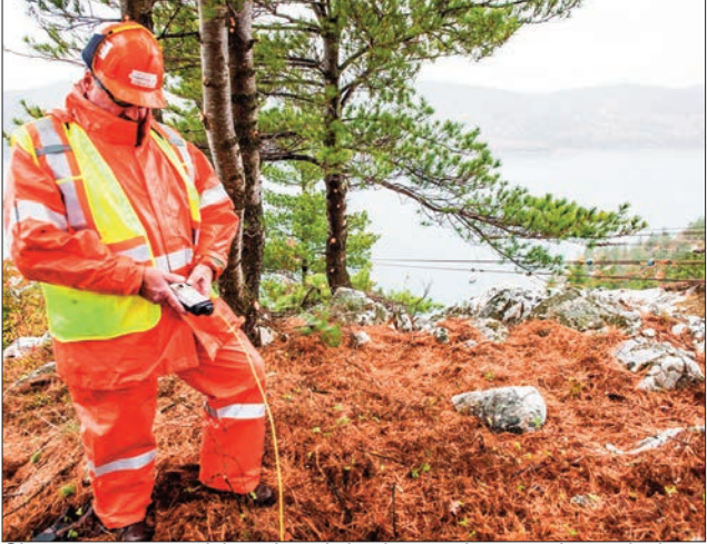
Charges are set and the primer is in place to detonate the explosives that will cut the lines supporting the Long Span.
