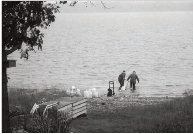
Jim Strong and Bill Caesar of White's Point submerge the Strong's water line with sandbags in the fall of 2012.
