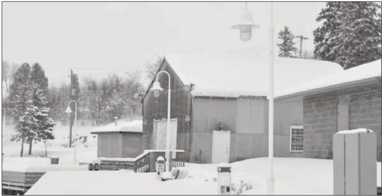
The OPP boathouse sits, in rough shape, on the new Little Current waterfront. The Northeast Town council hopes that the Ministry of Community Safety and Correctional Services, along with Infrastructure Ontario, enter the discussion to replace the deteriorating building.
