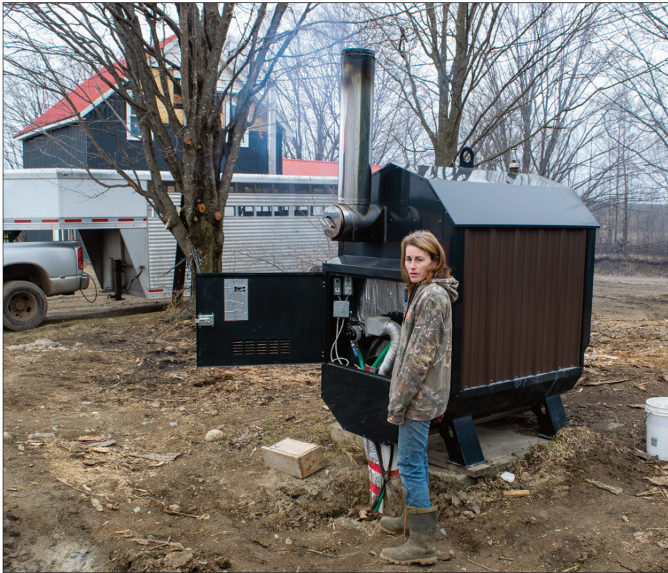
A wood-fired boiler has many purposes for the Pyette family. While one hose run supplies wintertime heat in the new greenhouse, another run is connected to the family home and provides warmth during the off-season.
