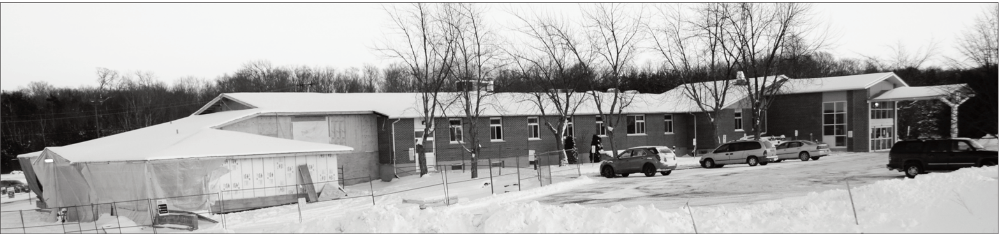
The 3,700 square foot building/addition of the Manitoulin Central Family Health Team (FHT) to the Manitoulin Health Centre, Mindemoya site, is well underway with walls, a roof and the cement floor poured as of last week. The FHT hopes to be in its new space by the spring.
