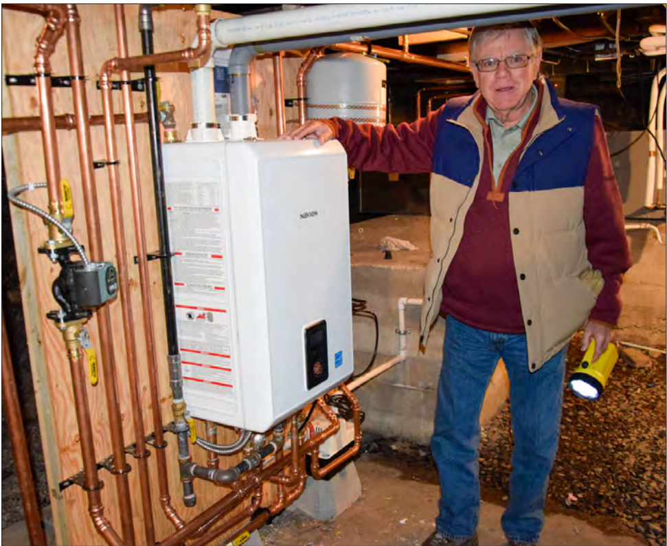
Little Current United Church Council Chair Scott Mosher stands by one of the hot water boilers that provides hot water to the coils within the forced air heating ducts.
