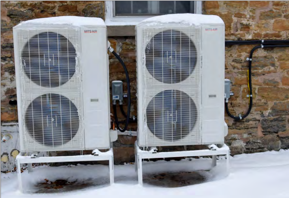
The twin heat pumps stand outside the church building in Little Current. One heats the main church building, while the other heats the hall.
