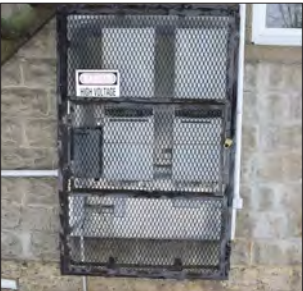
Control panels regulate the transfer of energy into the grid.
