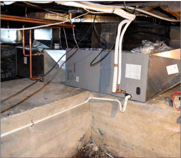
One of the two duct systems that heat the buildings. The massive slab is not subterranean pagan sacrificial altar but stood as a base for an old massive oil furnace.
