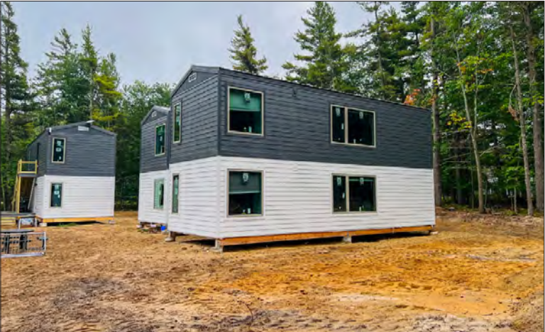
Modular housing units built on the mainland and taken to Beaver Island on barges.
